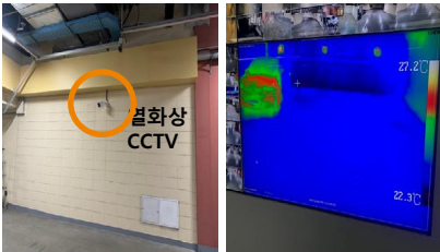
[Thermal imaging camera for electric vehicle fire response]
