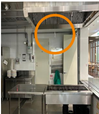
[Automatic fire suppression system for cafeteria]
